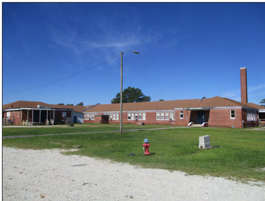
Photograph 12: View of the Back Hall's east elevation; looking west-southwest. (2018)
