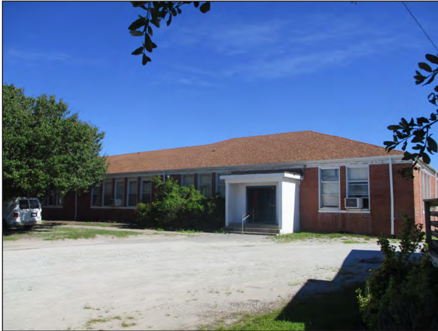
Photograph 15: View of Back Hall's south wing; looking north-northwest. (2018)
