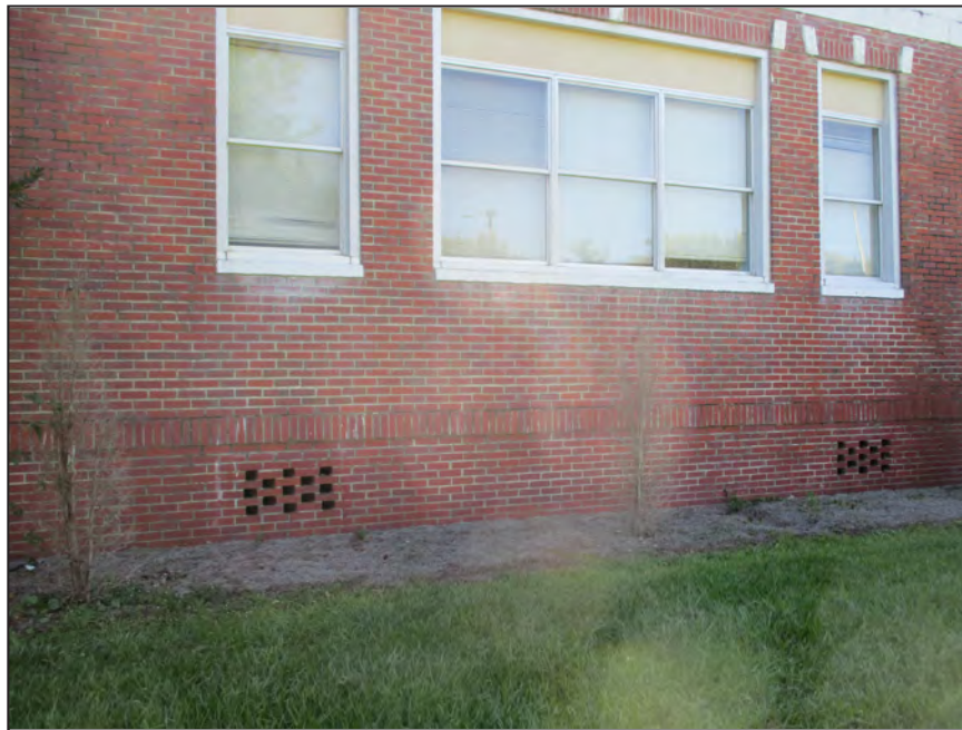
Photograph 3: Detail of water table on Dixon School's Front Hall; looking east. (2018)
