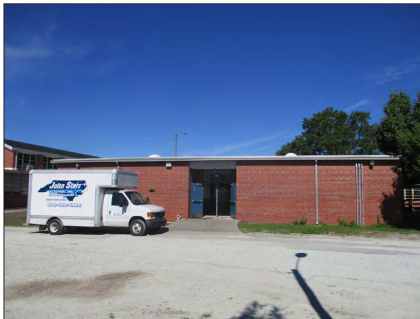
Photograph 29: View of Annex's east elevation; looking west. (2018)
