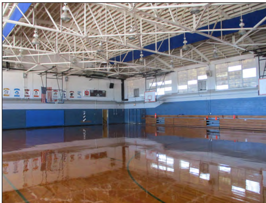
Photograph 28: Interior of 1953 gymnasium addition; looking southeast. (2018)
