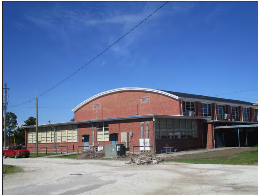
Photograph 24: Oblique view of gymnasium and band room; looking southwest. (2018)
