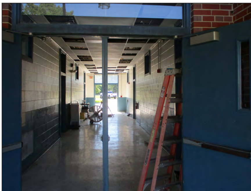
Photograph 30: Interior view of Annex; looking east. (2018)
