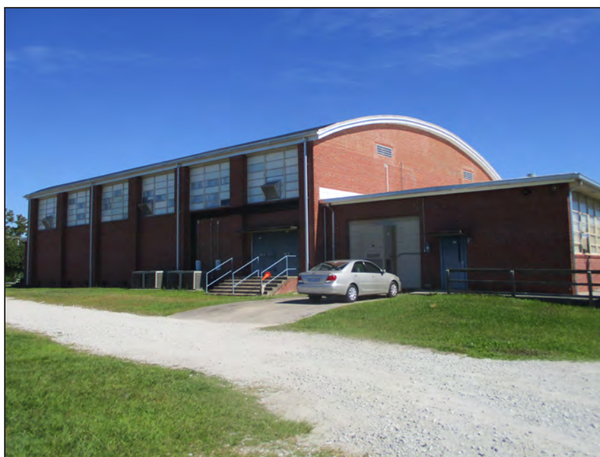
Photograph 23: View of gymnasium and band room's south elevation; looking northwest. (2018)
