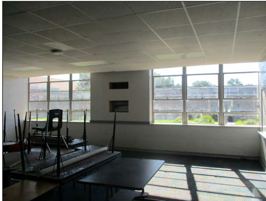
Photograph 26: Interior of 1953 classroom addition; looking east. (2018)
