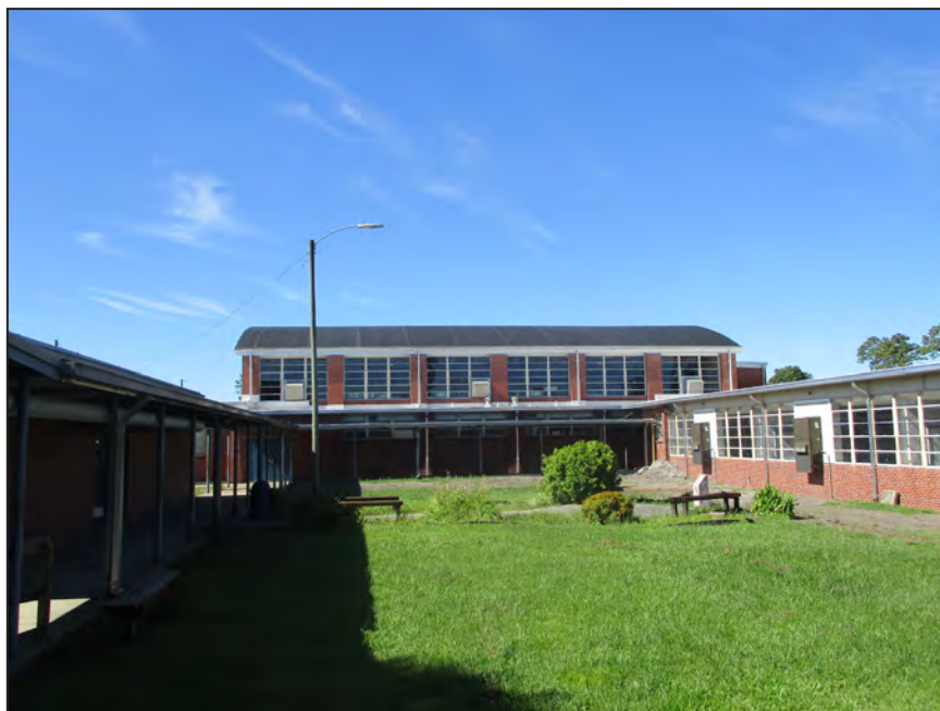
Photograph 25: View of gymnasium and north wing; looking south. (2018)
