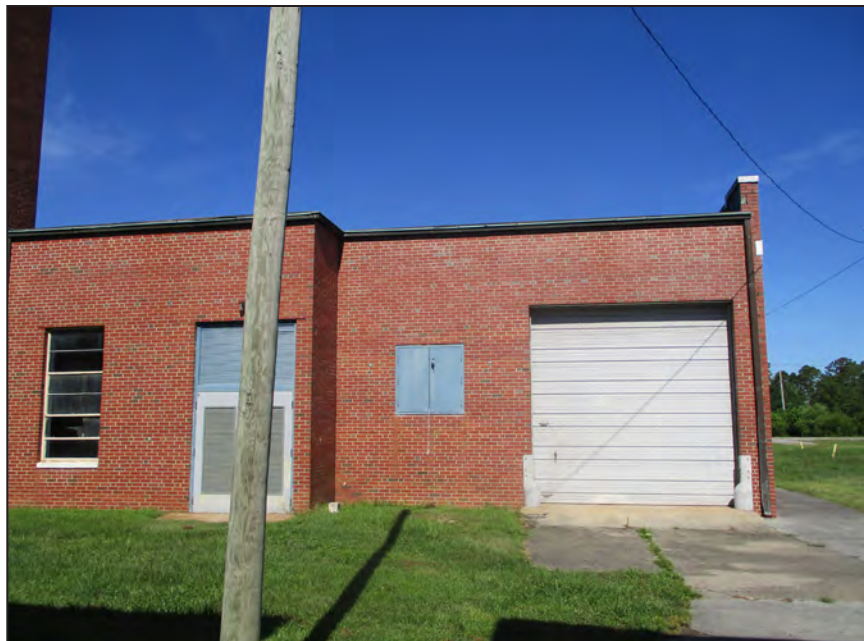
Photograph 8: View of boiler room's east elevation; looking west. (2018)
