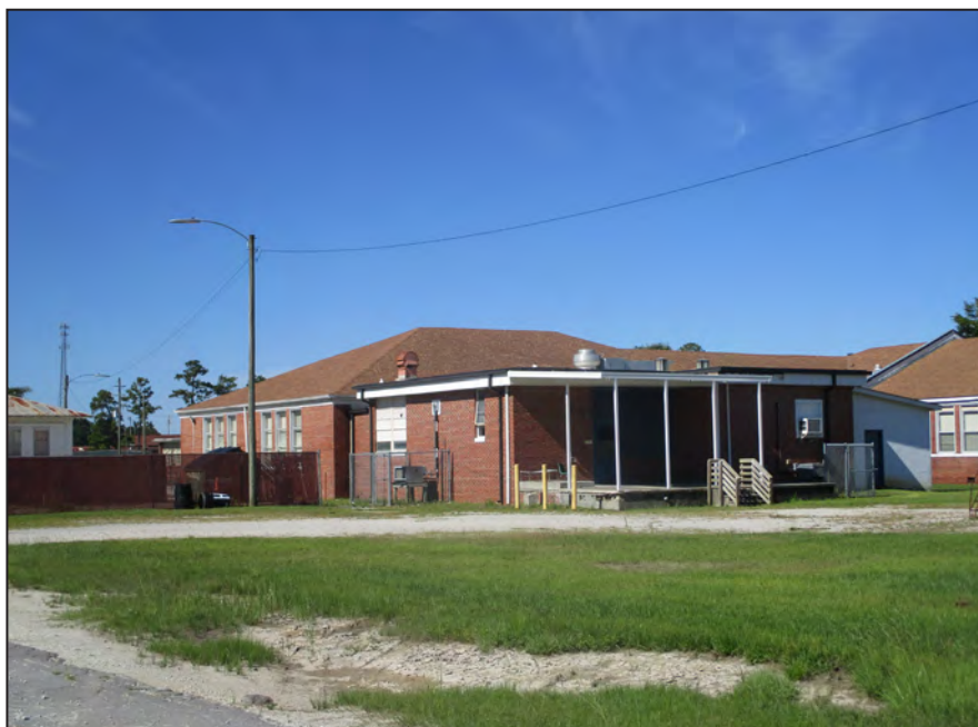
Photograph 14: View of Back Hall's south wing; looking southwest. (2018)
